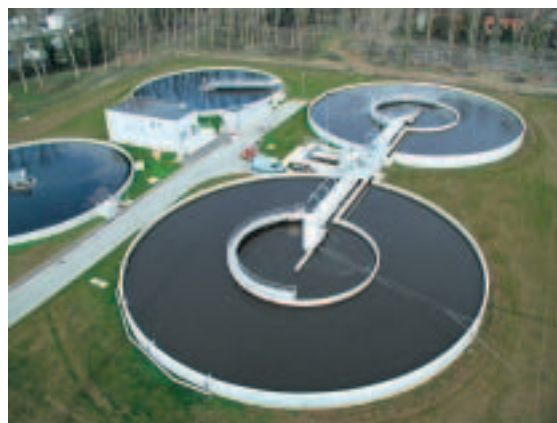
Photo 1 – Station d'épuration de Montauban (E. Cotteux, oct. 2000).
