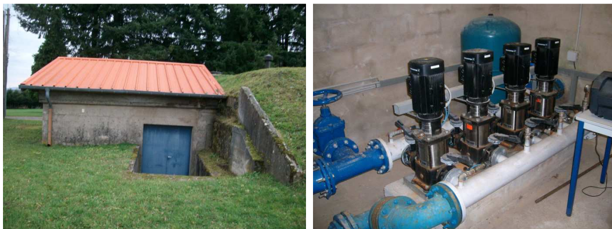
Figure 17: Photographies de la station de surpression
