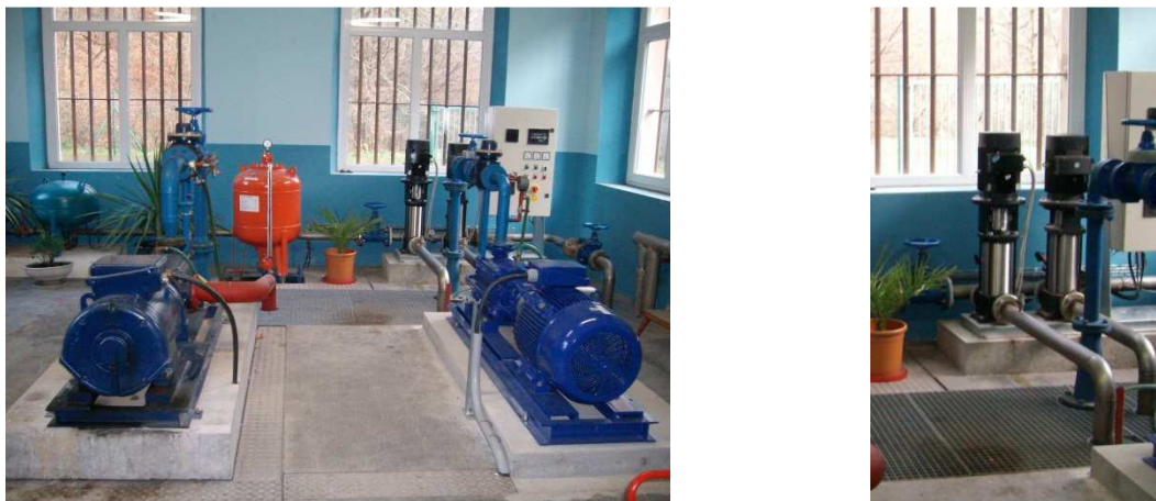
Figure 11: Photographies de la station de pompage
